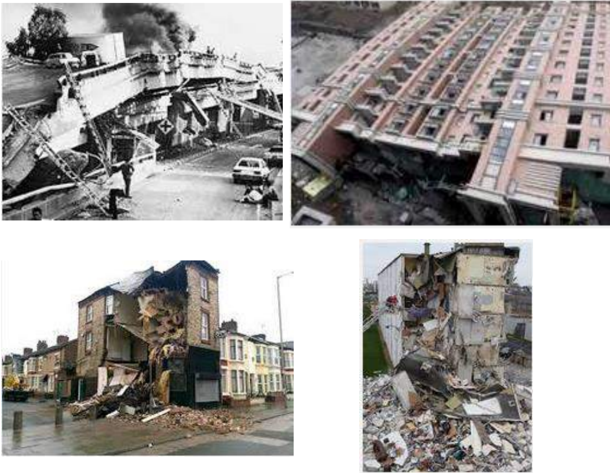
Fig. 2.1: The structure collapse
